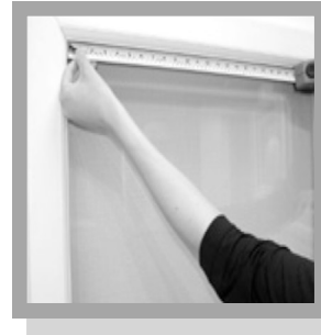
Step #2 - Measure Window Depth
