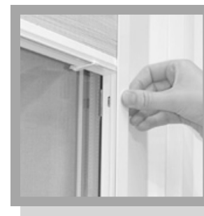
Step #2 - Attaching Frame to Window
