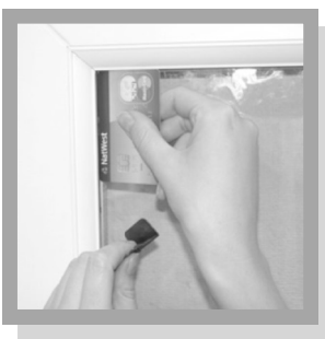
Step #1 - Insert Brackets
