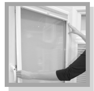
Step #2 - Attaching Frame to Window
