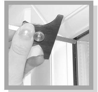
Step #2 - Measure Window Depth
